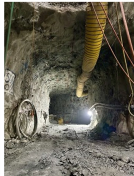
2. View North from shaft along Substation location
