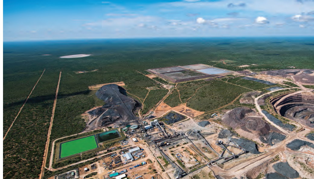
Aerial view of tailings (black color) and slimes (square containment)
