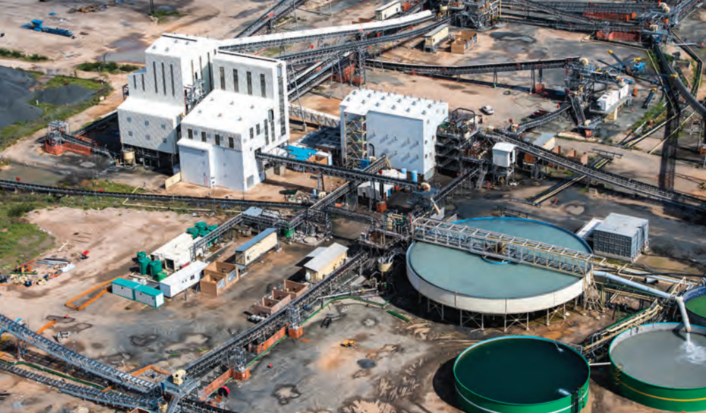
Aerial view of Karowe processing plant and water treatment plant
