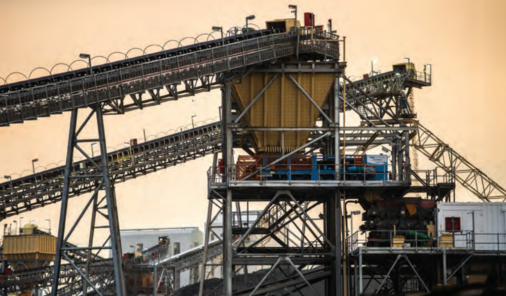
Conveyors and ore processing facilities
